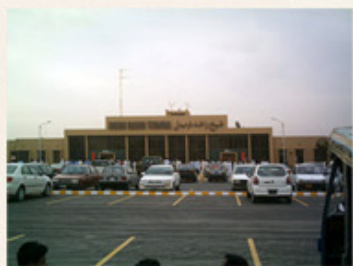
Sheikh Rashid Air Terminal
