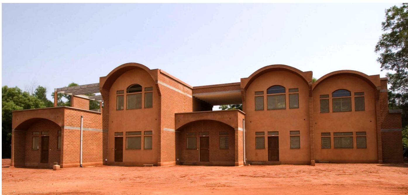
Figure 2: Apartments constructed with stabilized compressed earth blocks in Auroville, India 10
